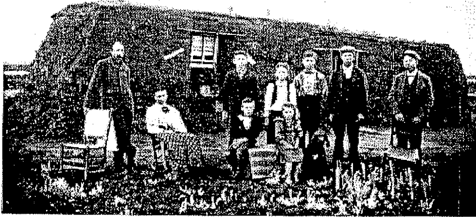
An unusually well built sod house of the Dakota prairies. Note the windows and doors providing comfort year round.
