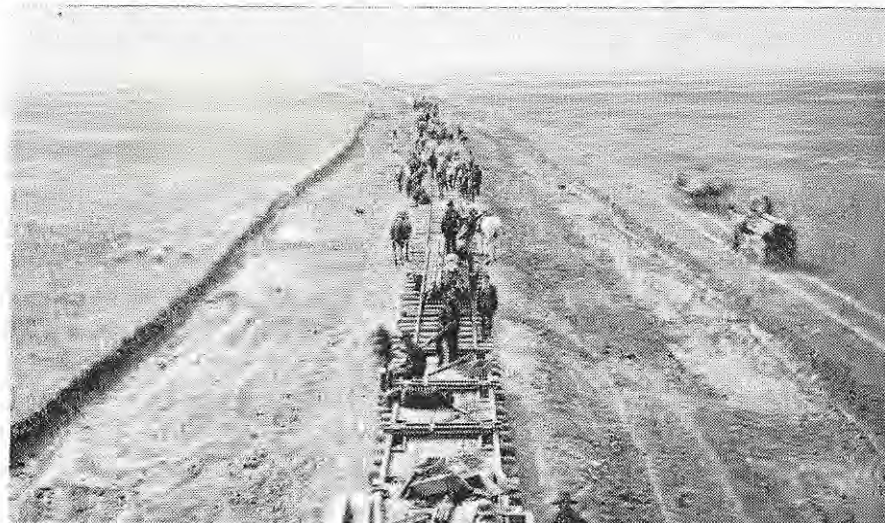
Constructing the railroad in the late 80's. Material train brought the rail, ties and other supplies to within a short distance of the rail head. Iron cars, drawn by horses, moved the rails to the end of the track, while teams went ahead with ties and the timber for bridges.
