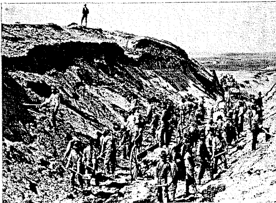
In 1879 Northern Pacific grading crews were busily constructing right-of-way through Dakota Territory. This picture shows the Big Sand Cut, Sweet Briar Valley. — Photo through the courtesy of Haynes Studio, Bozeman, Mont.
