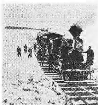
Taken on Feb. 12, 1879, the above picture shows an N. P. train crossing the Missouri River between Mandan and Bismarck on rails laid on the ice.
